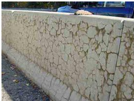
Figure 1: Characteristic AAR: Pattern Cracking
